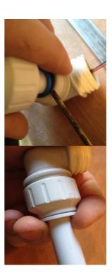
D. Screw on the cap till tight then release with half a turn, and very slowly squeeze the pipe in holding the release washer as you go. You will feel the pipe seated. Cut the pipe to your desired length.
